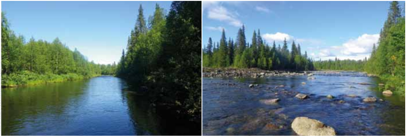
Before and after photos showing the addition of gravel and boulders to improve the quality of fish spawning sites on the Vindel River
