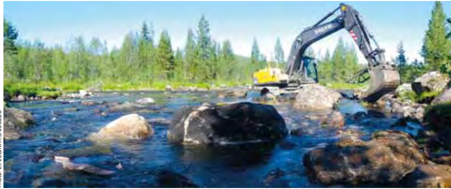
Dr Johanna Gardeström: “Large structures... are especially important during high water conditions to prevent smaller materials being flushed away.”
