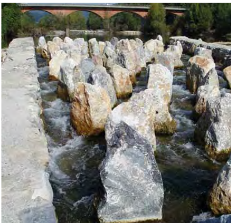
Fish pass near Sarzana railway bridge. The project found that sea lampreys prefer passes with boulders in a grid pattern
