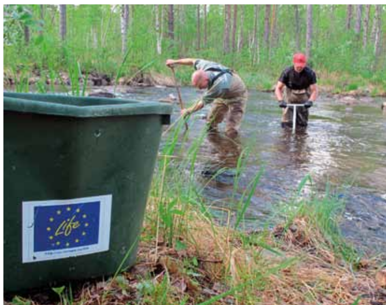
River restoration work in progress (June 2011)
