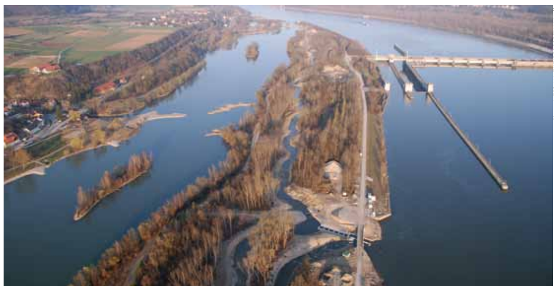
Aerial view of the 2 km-long fish pass constructed by the Donau-Ybbs project
