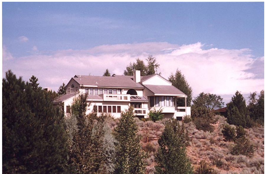
Figure 3—Planning is the first step to making a home site in the wildland-urban intermix safe from wildland fire.
