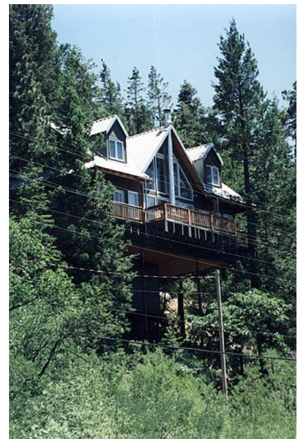
Figure 12—Power lines can be a safety hazard in the wildland-urban intermix.
