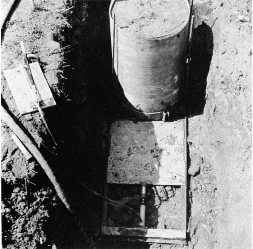
PLATE 2. Insertion of the steel cutting plate under the lysimeter casing.
