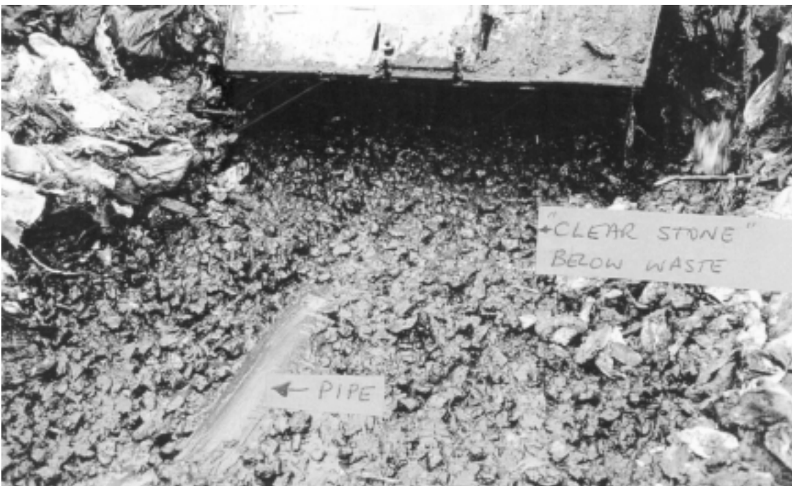
Fig. 10. Exhumation of temporary toe header at KVL.
