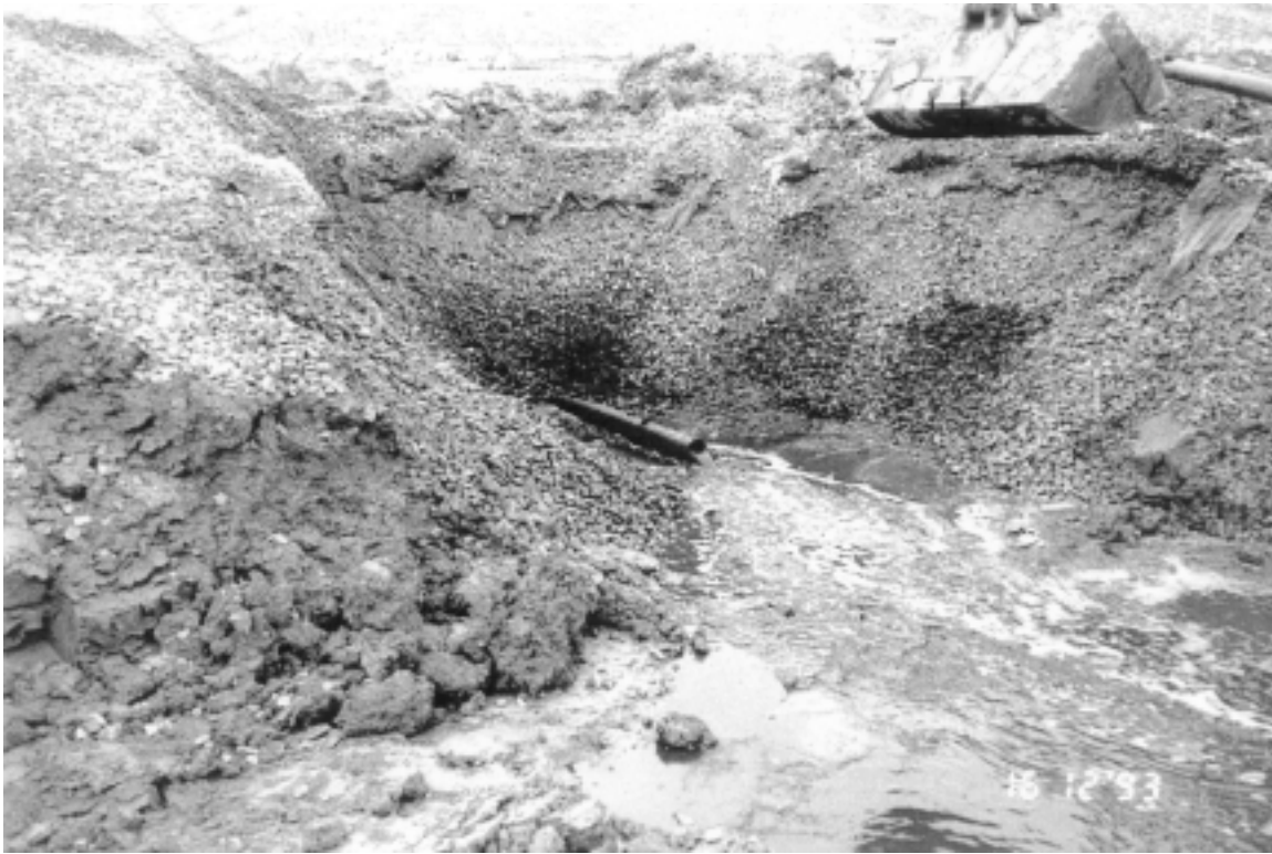
Fig. 12. Exhumation of temporary collector pipe (1993).
