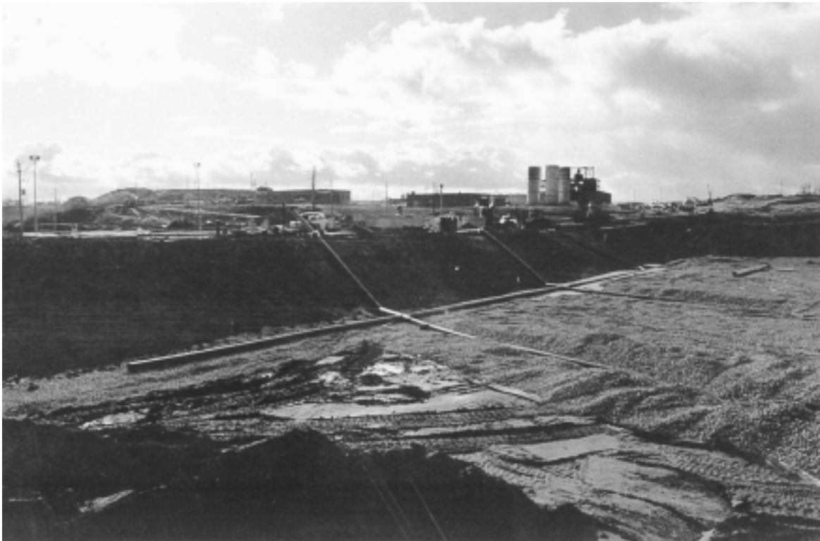
Fig. 8. Clear stone drainage layer at Keele Valley.
