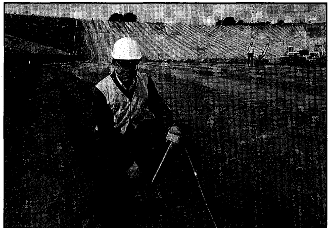
Photo 2. Electrode and geophysical cable installation.
