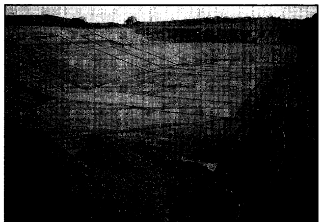
Photo 1. Shallow trench lines for the geophysical cables map out the position of the grid during landfill.
