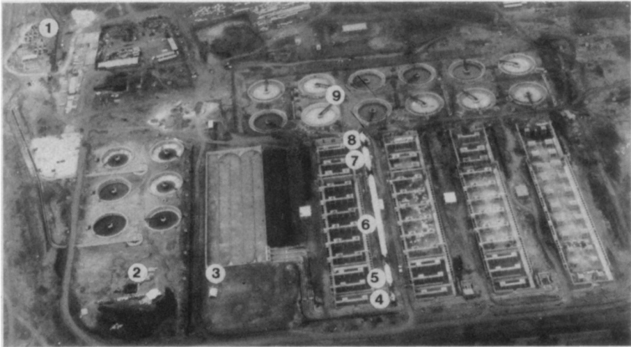
FIGURE 11. The 150 000-m 3 /d Johannesburg Goudkoppies Works under construction in 1977. (1) coarse and fine screens, (2) primary sedimentation tanks, (3) balancing tank, (4) anaerobic zone, (5) primary anoxic zone, (6) primary aeration zone, (7) secondary anoxic zone, (8) secondary aeration zone, and (9) final clarifiers.
