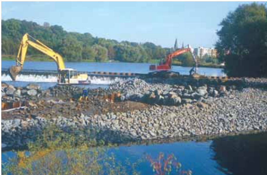
Figure 4.40: Spillenburg weir; fish ramp under construction
