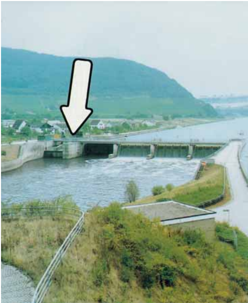
Figure 5.44: The Schoden/Saar fish lock (view of the weir installation)
