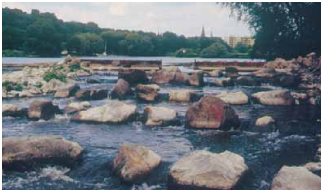
Figure 4.41: Spillenburg weir; fish ramp after completion
