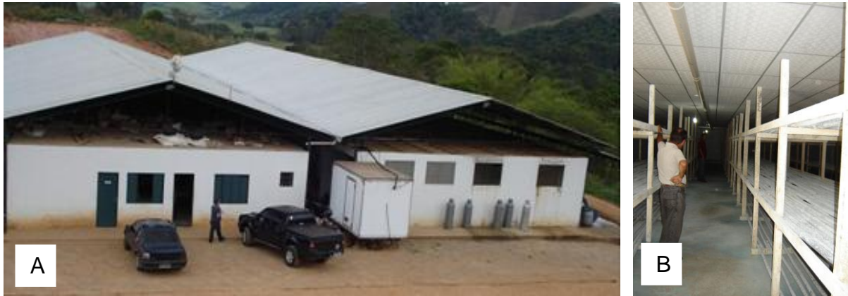
Figure 4. A: Modern production buildings with environmental control in the mountainous region of Mata Atlantica. B: Internal view of a growing room that has thermal insulation and wooden benches containing 3 levels. Each room is 25 m long, 7 m wide and 3 m high.
